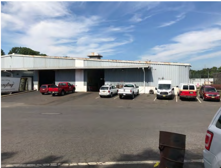
East Side Warehouse & Auto Shop Drive - In
